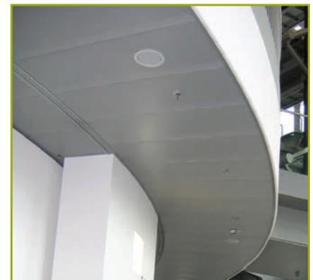
**Figure 7:** Passive beams installed behind a metal perforated ceiling
