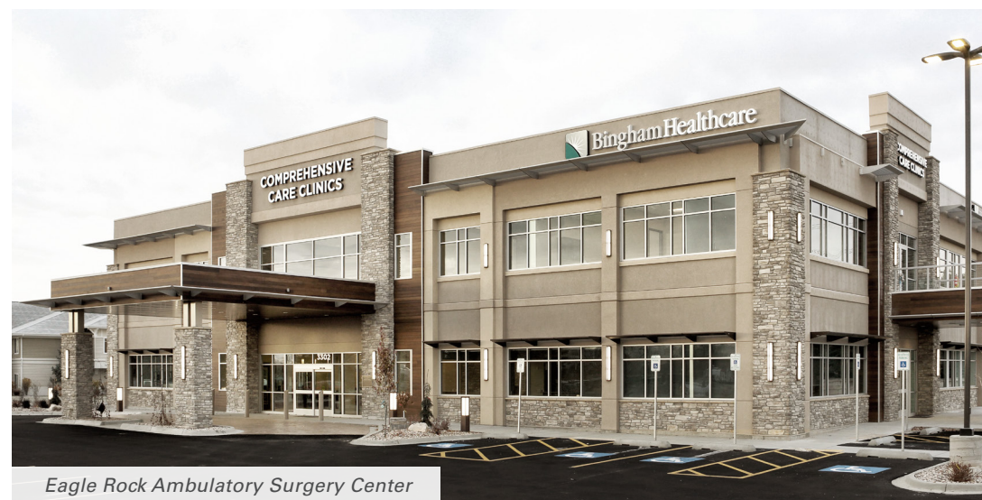
Ultrasuite installed at the Eagle Rock Ambulatory Surgery Center
